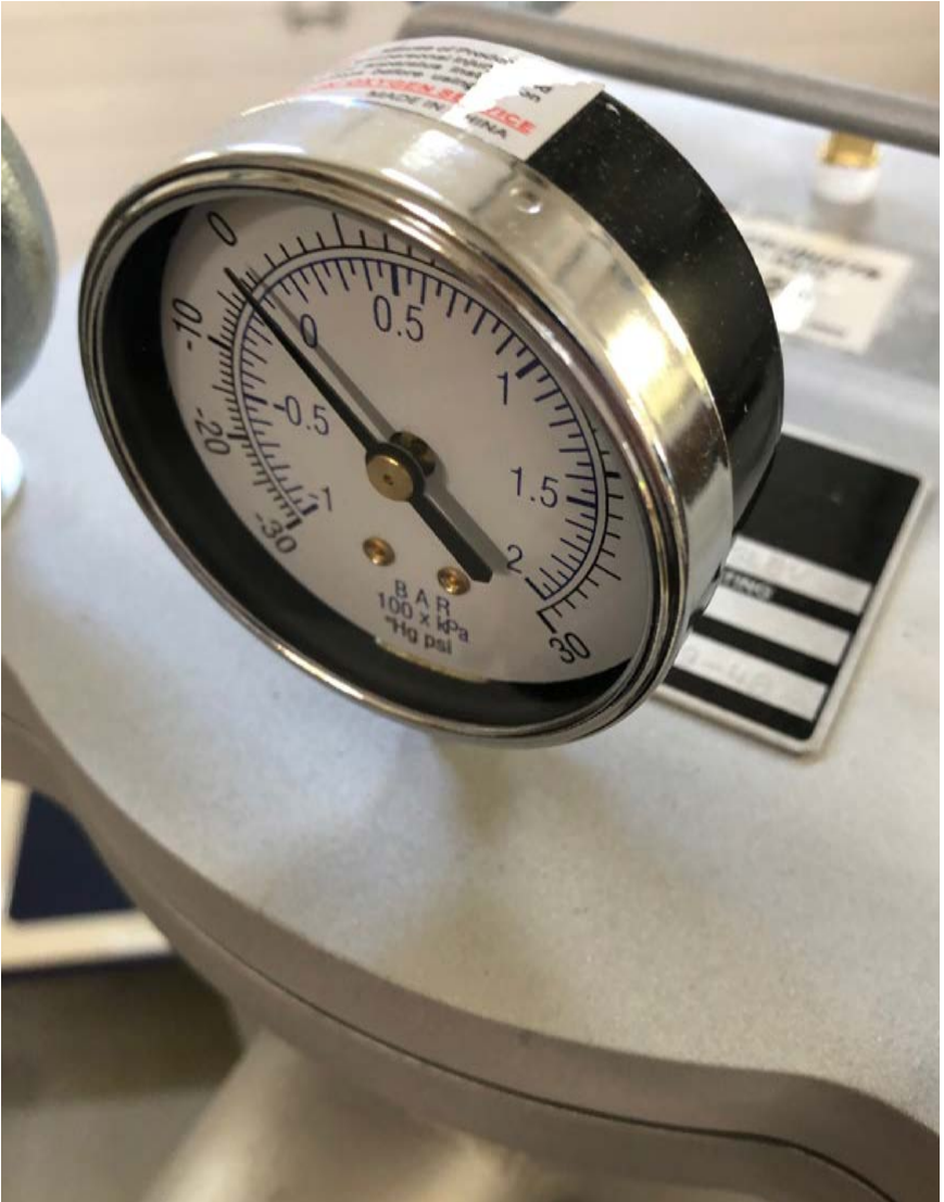
Inlet Vacuum Gauge Installed
